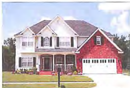
examples of ill proportioned windows with shutters
