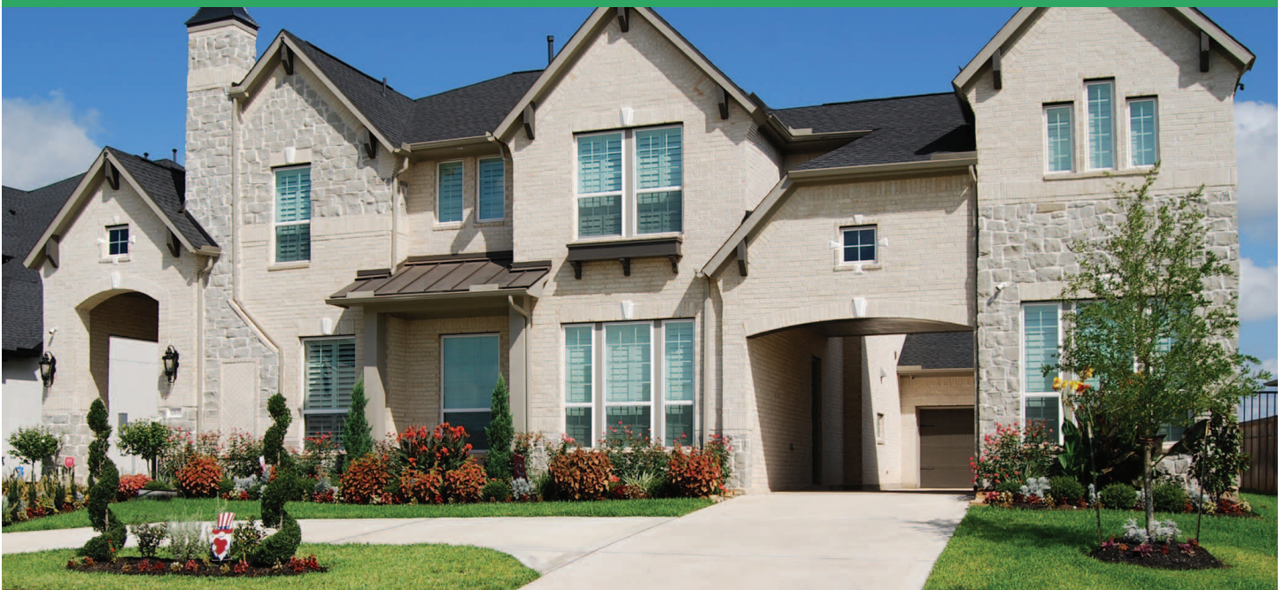
FRONT ELEVATION OF DWELLING
