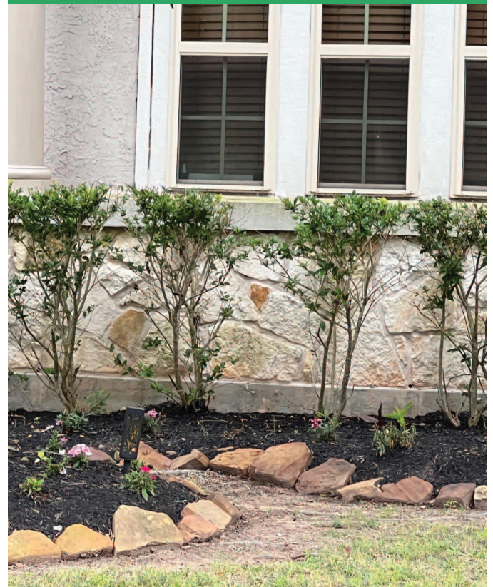
FOUNDATION SCREENING VIOLATION - 'LEGGY' SHRUBS
