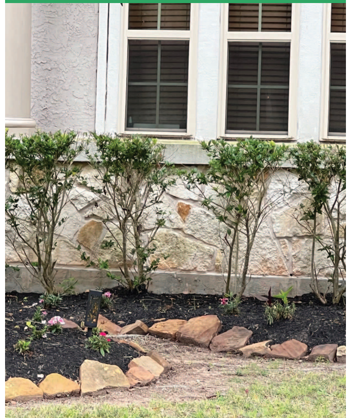
FOUNDATION SCREENING VIOLATION - 'LEGGY' SHRUBS
